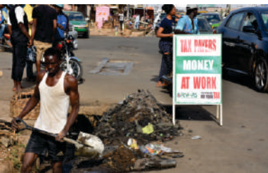
Clearing of Drainage
