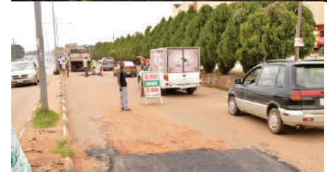
Patching of Tanke Road, Ilorin
