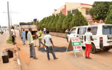
Patching of Tanke Road
