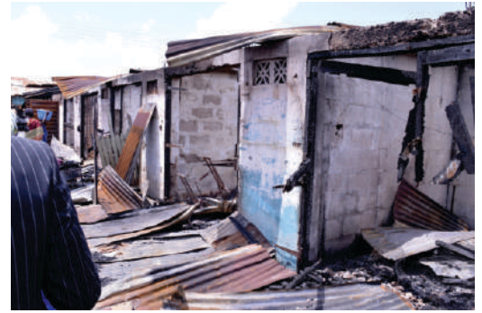
BEFORE (The Renovation of 40 burnt shops at Baboko)
