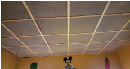
Fixing of Children Specialist Hospital Ceiling
