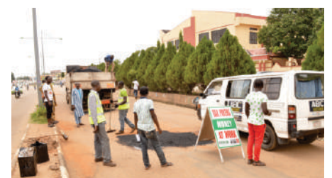
Patching of Tanke Road, Ilorin
