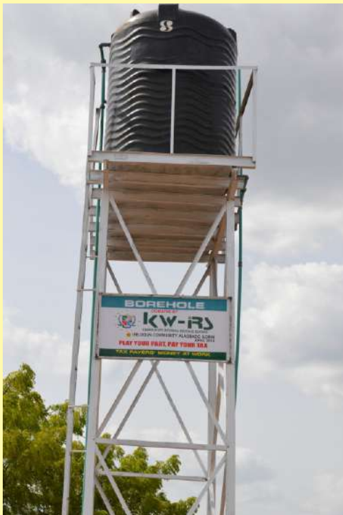
KW-IRS donate borehole to Alagbado Community
