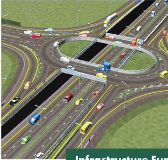
Gerik-Alimi Split Diamond Underpass
