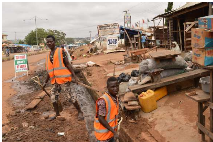
Clearing of drainages
