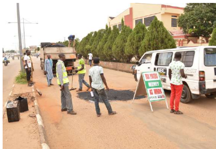
Patching of the road for smooth movement
