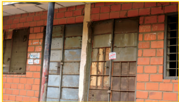
A shop under lock by KW-IRS
