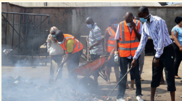
Environmental clearing & cleaning
