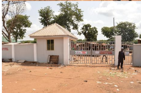
Kara Market fencing and Gate House
