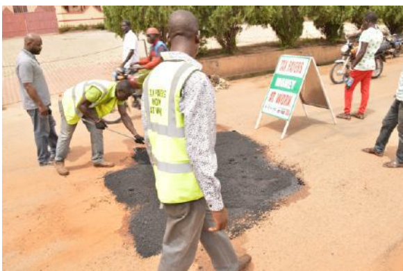
Patching of Tanke Road
