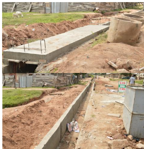
Construction of drainage in Kaiama
