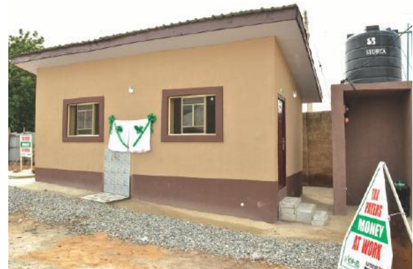
Construction of Public Toilet at Ago Market
