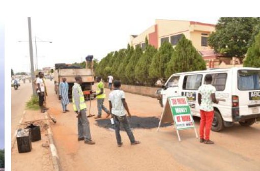
Patching of Tanke Road
