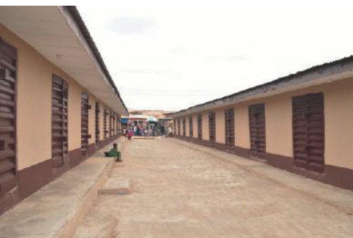
40 Shops constructed at Oja Tuntun
